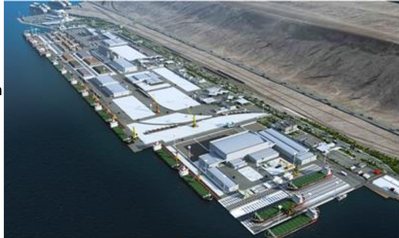
Turkmenbasy International Sea Port Project
